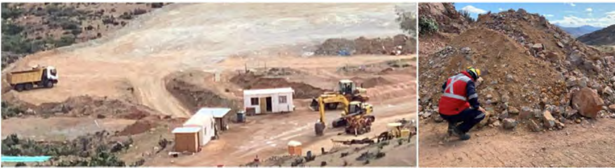
Figure 17 First Mining at Santa Innes Underground Mine, Productora project
