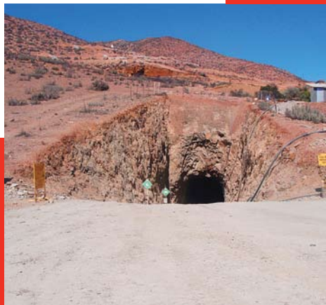
Productora underground mine portal
