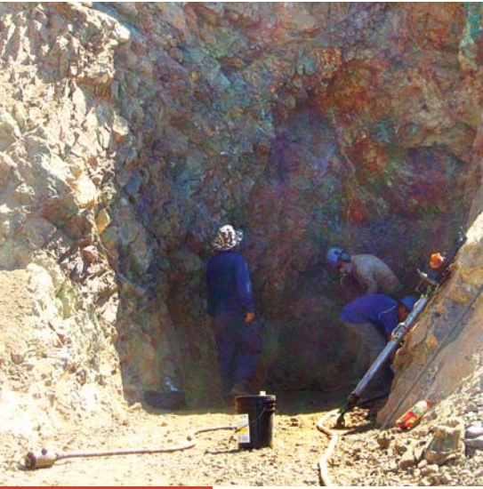
Surface blasting crew at Los Mantos
