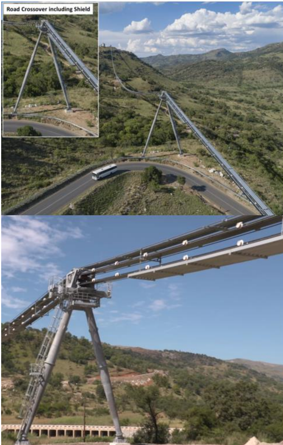
Figure 18.22 Rope Conveyor installation example including shielding plates above roadway
